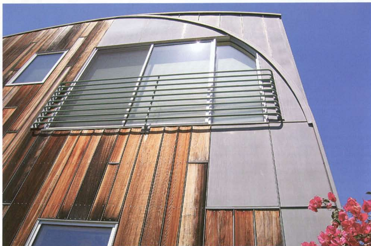
The exterior is clad in redwood from old Northern California wine vats and zinc sheeting.
